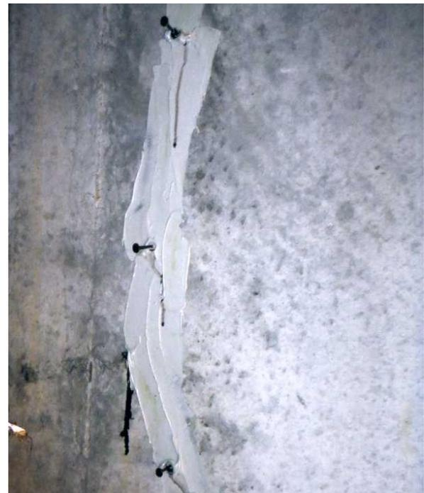
*A basement crack repaired with the injection of an epoxy material. Repairs such as this usually come with warranties against future movement along the repaired area, but not against cracking in other locations.*
