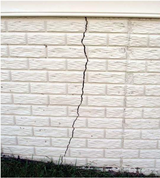
*This crack is wider at the top and extends all the way through the wall, allowing water intrusion. Professional repair is recommended.*
