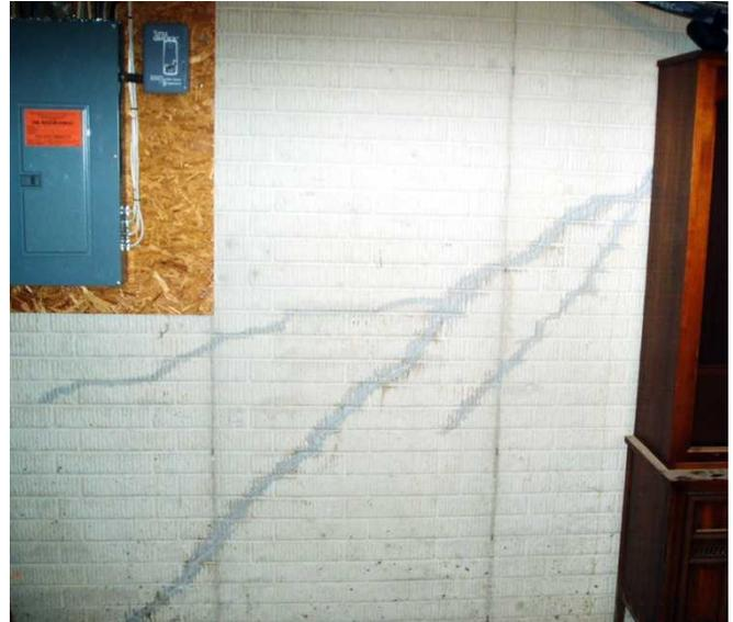
*Cracking due to settlement. This crack has been repaired, but should be monitored periodically for any future movement.*
