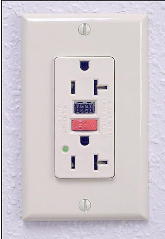
*A typical receptacle-type GFCI outlet. Note the TEST and RESET buttons*
