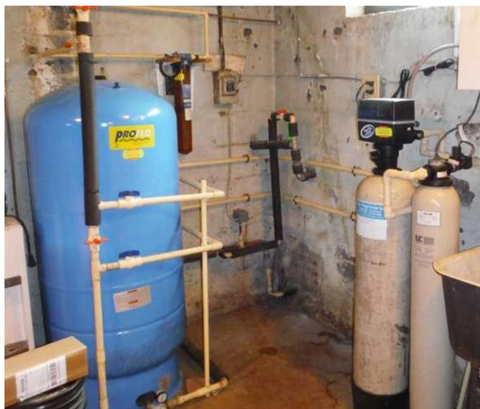
*Well tank and treatment system. Water enters the house and is stored in the 119-gallon pressure tank. It then flows through a cartridge filtration unit, neutralizer, and UV sterilizer.*
